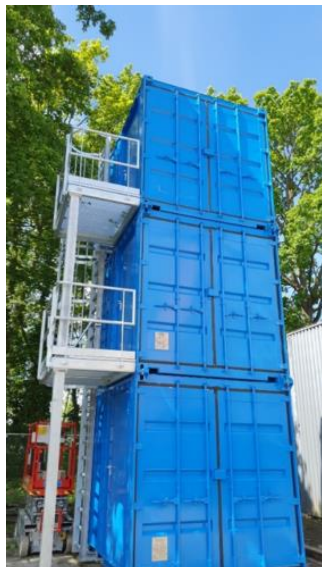
Fig. 1: TNO's small-scale ATEX-compliant mobile pilot plant
